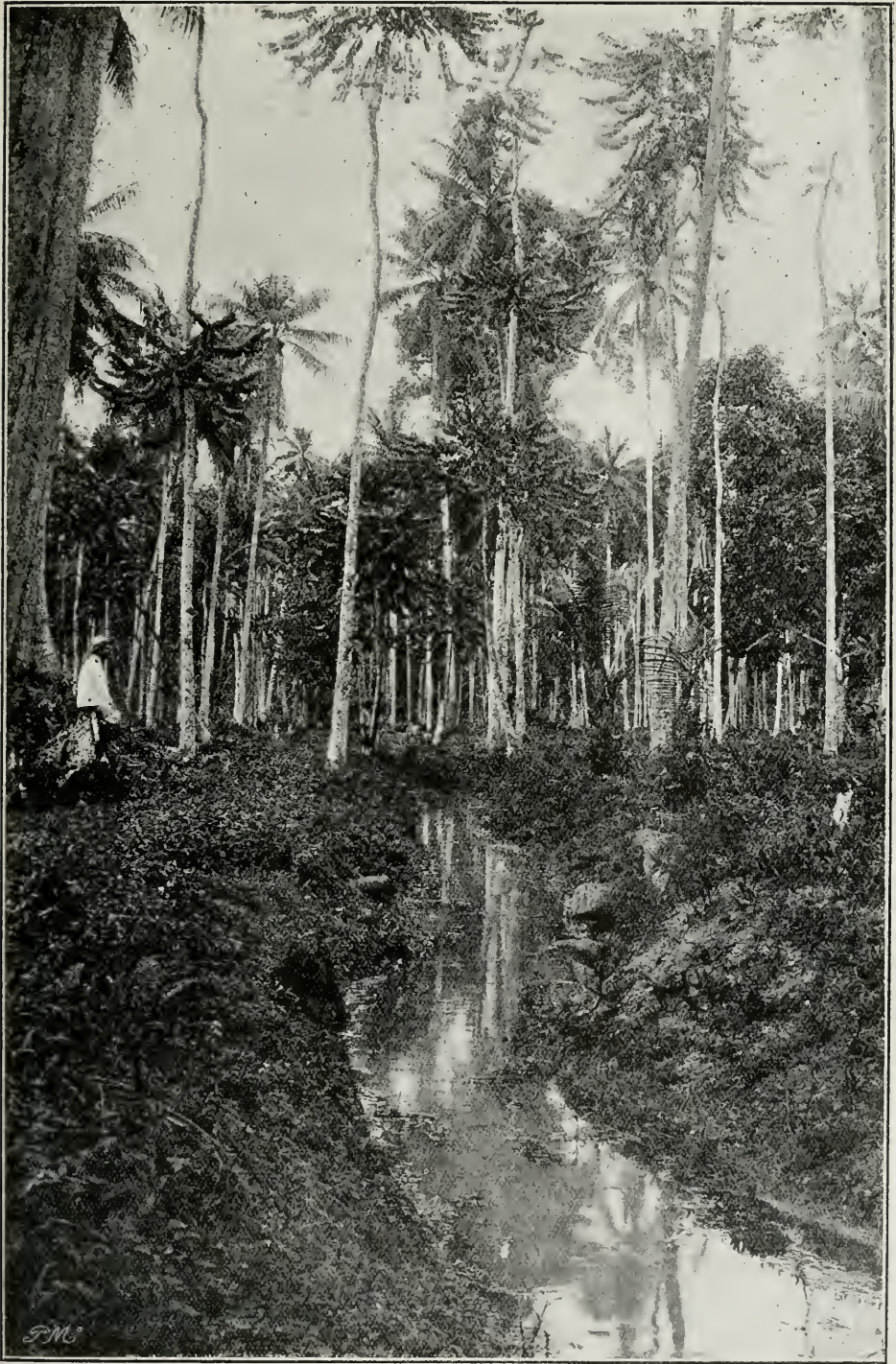
FIG. 33.—OUTFLOW DRAIN OF RIBEIRA GALLINHA, ROÇA PORTO-REAL.
